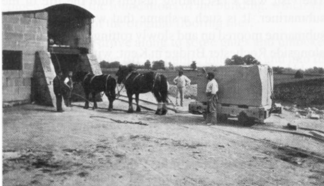
A block of stone is being prepared for transportation to Corsham station c. 1912. The winding engine house is seen on the left. Photo Nick McCamley collection
